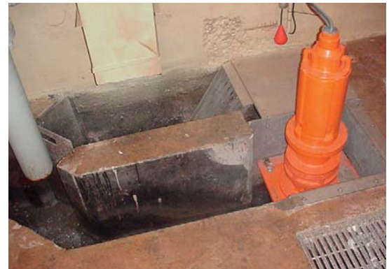
Grind Hog™ 16ASX T/S (3.5 mgd) installed
