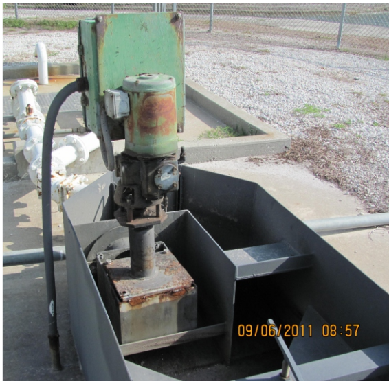
REPLACING ORIGINAL CLOW A-8
