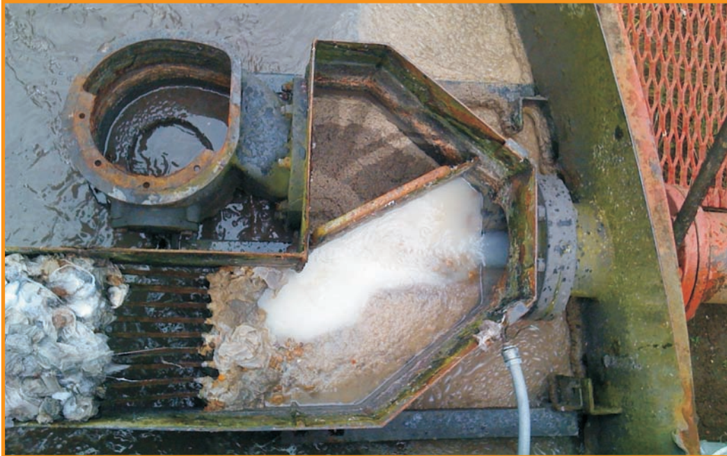
WORTHINGTON MODEL 7 & EXISTING SPLITTER BOX
