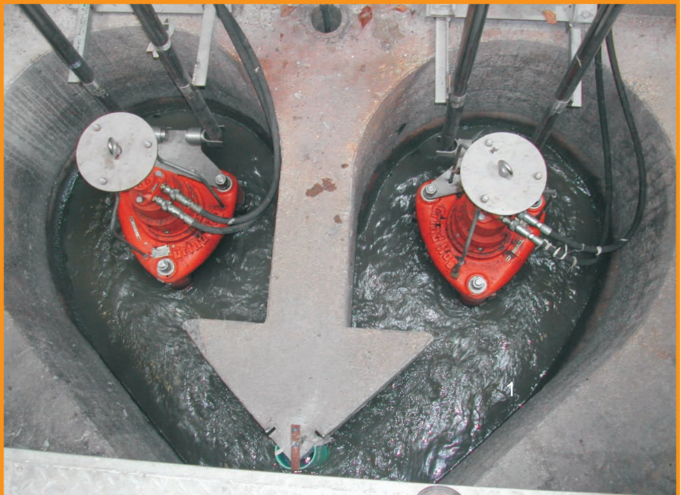
Replacing Chicago Pump Model 10C
