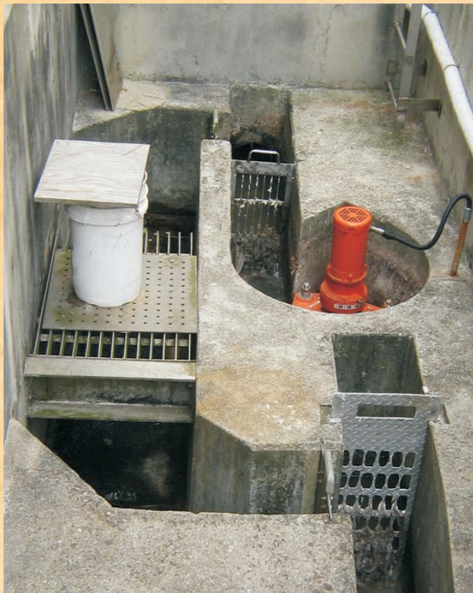
Using Existing Channel Installed GRIND HOG™ 10L
