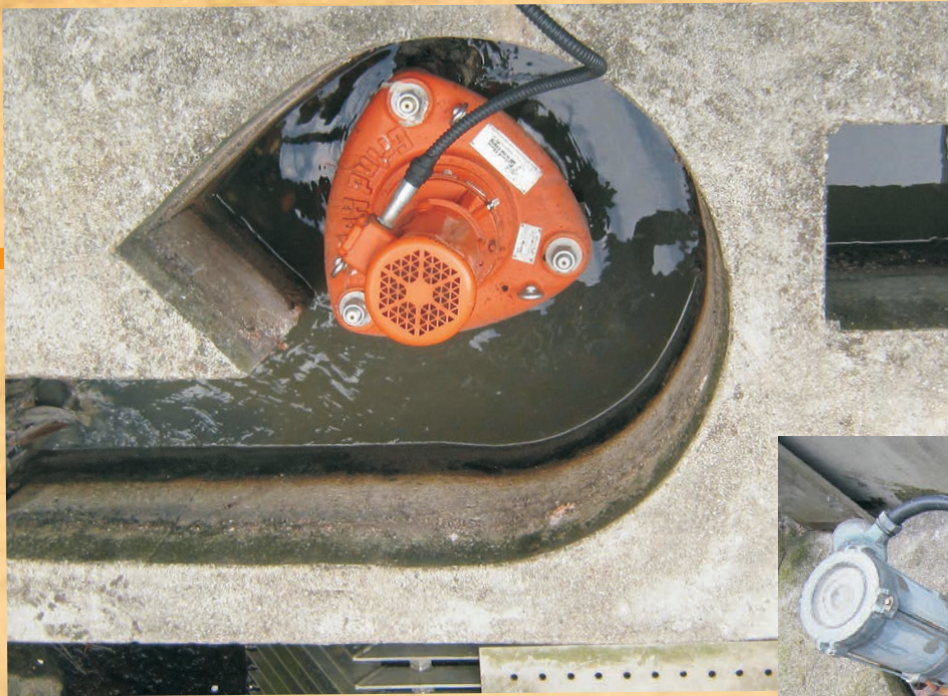
Using Existing Channel Installed GRIND HOG™ 10L
